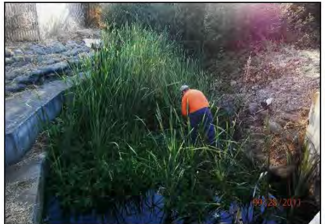
Photo 6. Sediment with vegetation growing on top of it in Belmont Creek at Old County Road. (September 2011)
