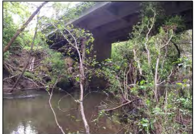
Photo 4. Pescadero Creek Road bridge near Cloverdale Road that requires routine maintenance including scour and erosion protection improvements at the base of the abutments. (April 2017)
