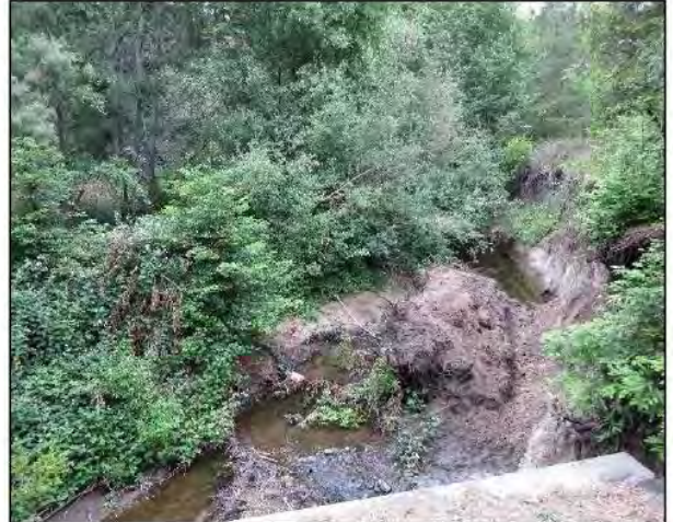
Photo 2. Example area that underwent hazardous tree removal in La Honda Creek (near Entrada Way). Photo shows mass of soil and redwood roots in middle portion of channel. (May 2015)
