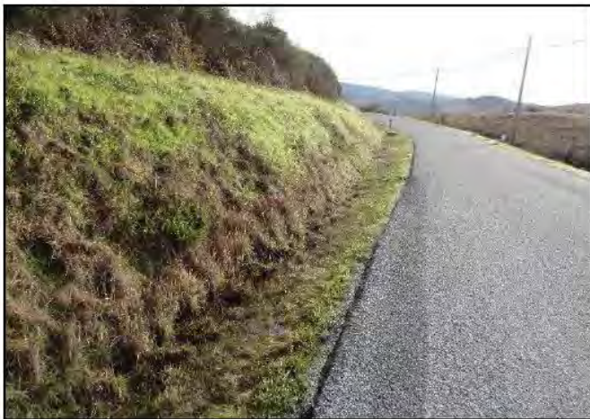
Photo 15. Example of an inboard unpaved ditch along Bean Hollow Road. (December 2019)
