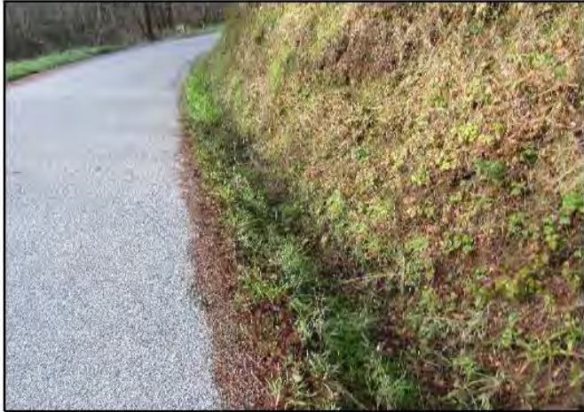
Photo 13. Example of an inboard unpaved ditch along Gazos Creek Road. (December 2019)
