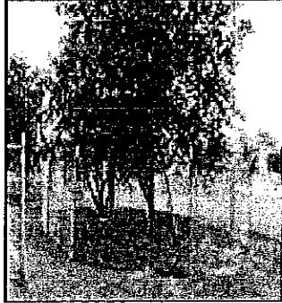
IMAGE 2.15-1 Tree Protection Fence at the Dripline
