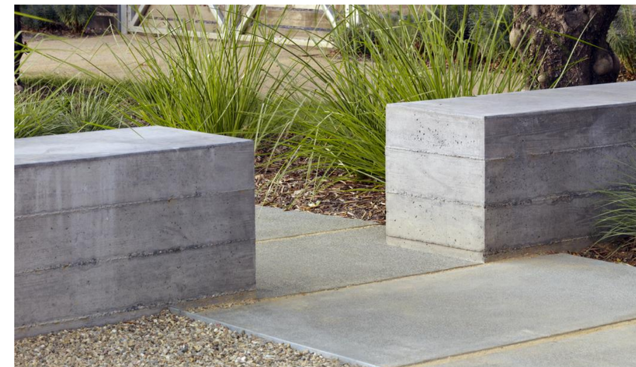
LANDSCAPE WALL AT DRIVEWAY (HORIZONTAL BOARD FORM FINISH)
