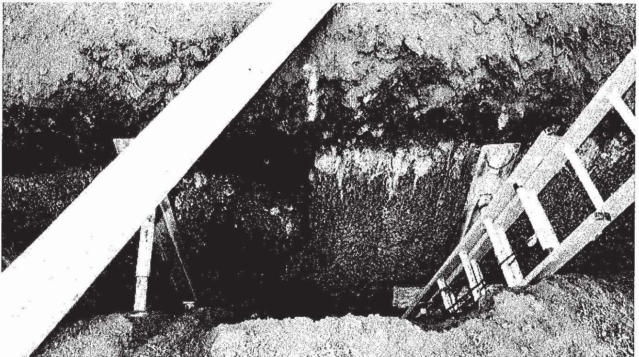
View of fault trace, north wall.
