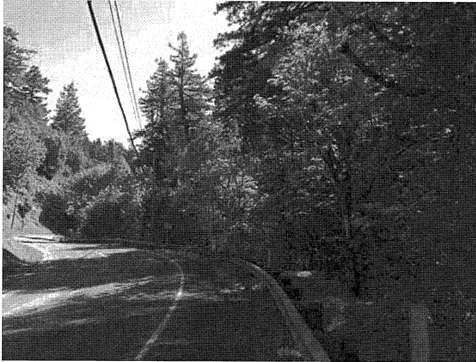
Photograph 3 View north of proposed Node 049A site.
