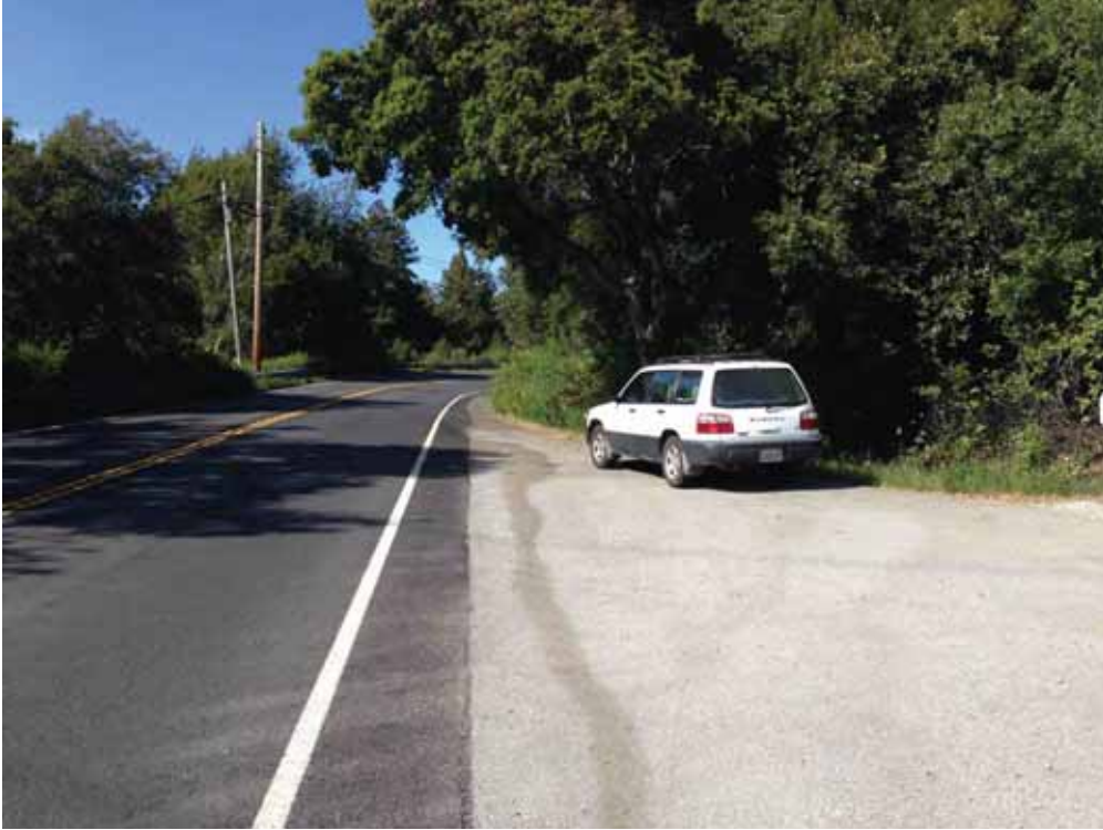
7: Node 057A Area Overview (North)
