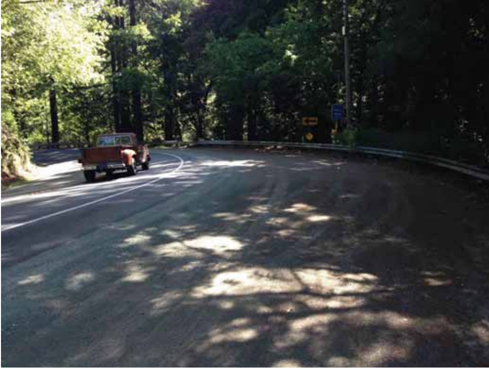
Photo 5: Node 050A Area Overview (South)
