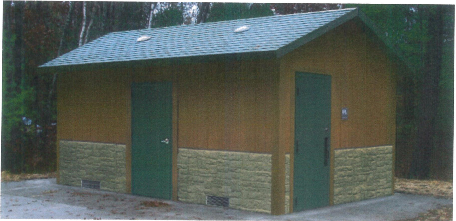
**Precast/Preassembled Reinforced Concrete Bathroom**
