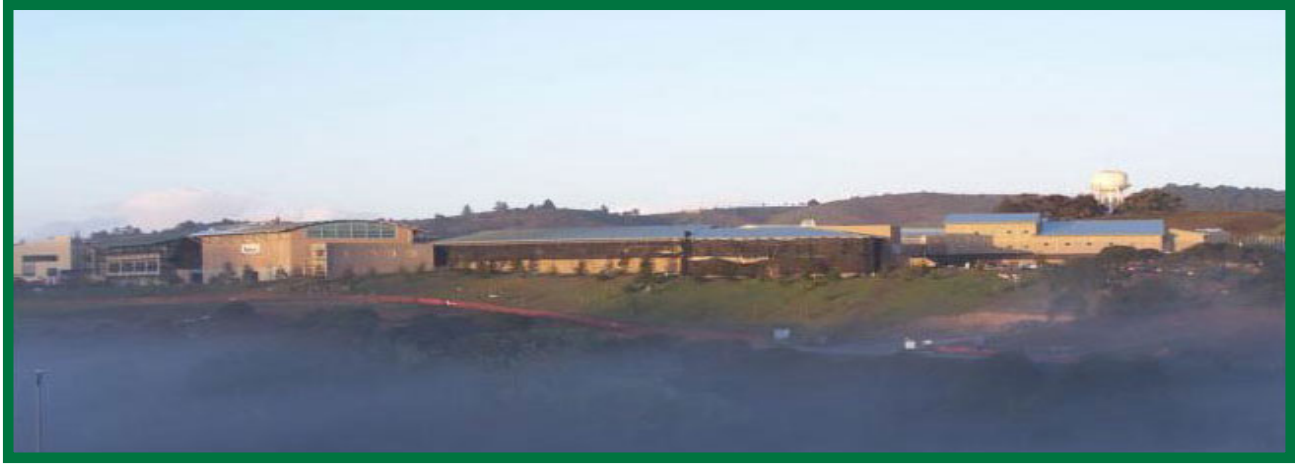
Newly Constructed Youth Services Center
