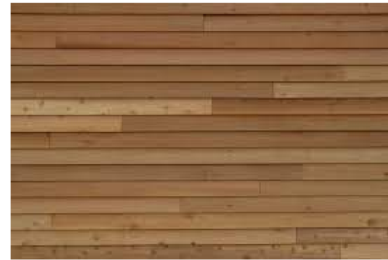
EXTERIOR WOOD SIDING FINISH
