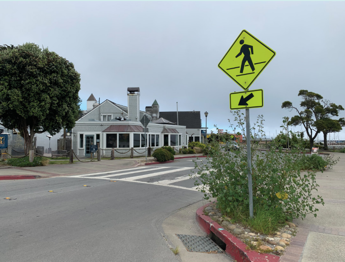
Curb extension and crosswalk in Princeton
